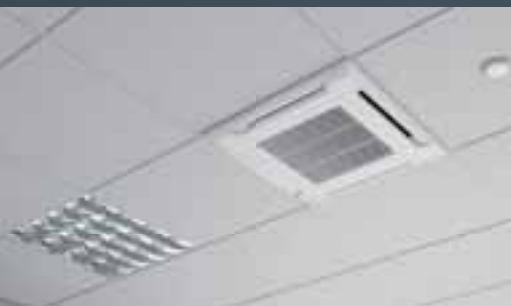
Compact Cassette Grid Type for VRF system: This fits grid ceiling system.
