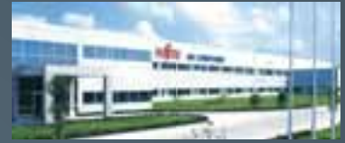
Fujitsu General (Shanghai) Co., Ltd.
